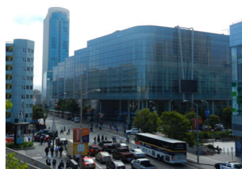
Moscone Center West Hall と Inter Continental Hotel (奥の細長いビル)
